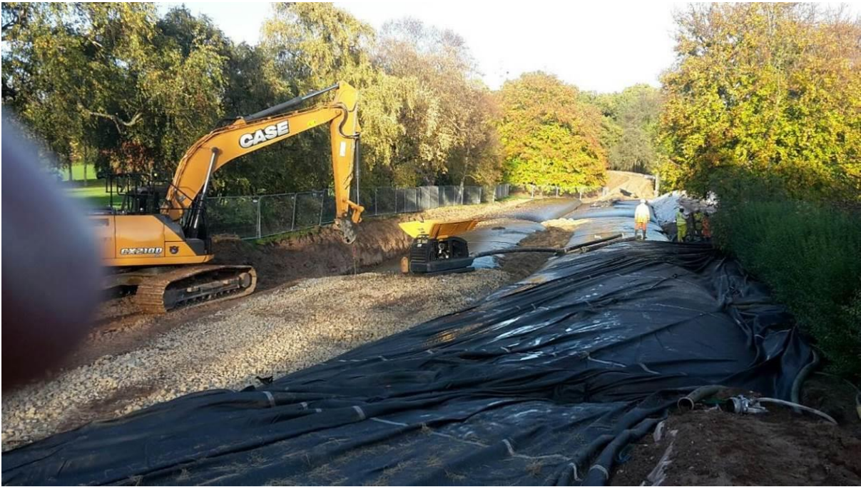
Geotubes full of silt
